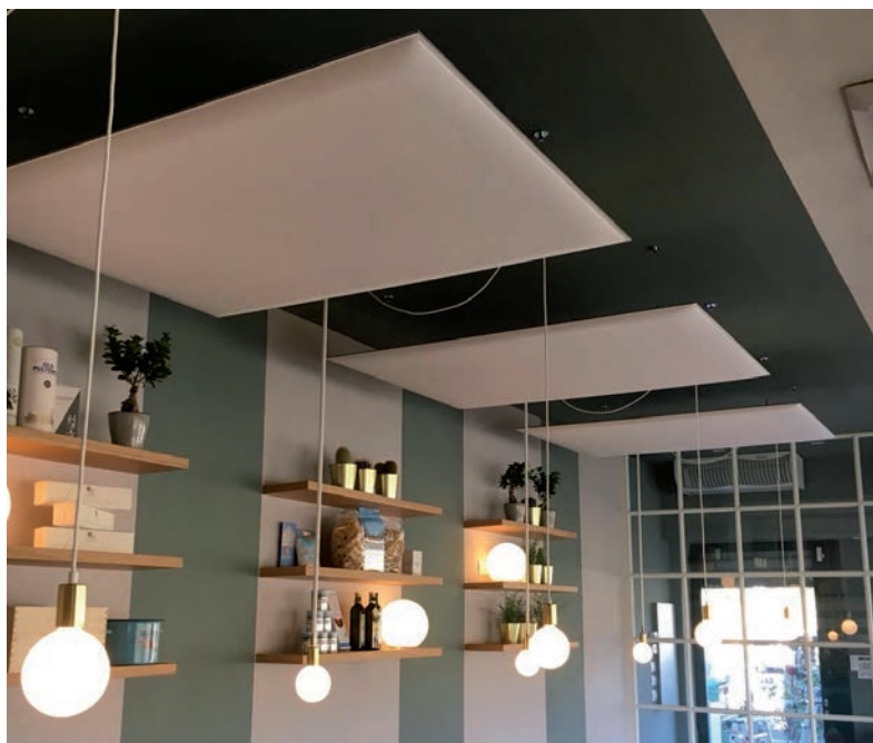
L'Amo, Arezzo (Italy) Snowsound ceiling, pannelli fonoassorbenti sound-absorbing panels
